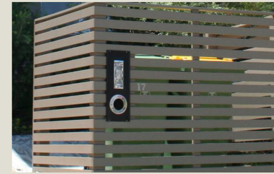
2.9 Bins at frontage and screened with fencing
