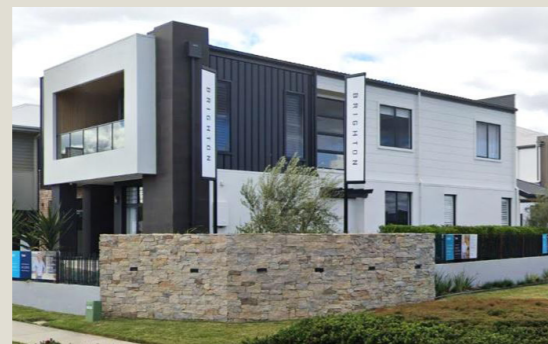
2.7 Window within 3m of front façade, Grd level and 2nd level defined through a combination of materials and articulation, material changes along the façade, windows to habitable rooms.
