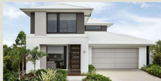
Use of articulation and colours to differentiate first and second floor (Image Source: Plantation Homes)
