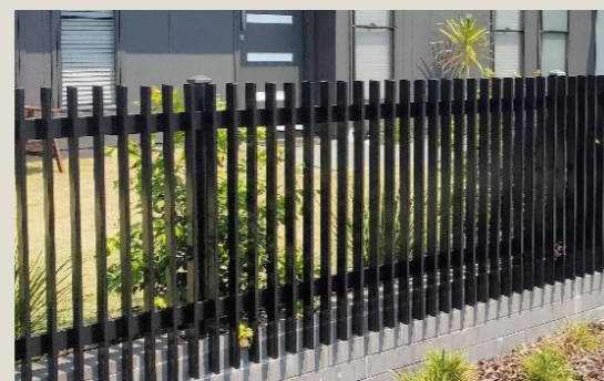
3.4.1 Spacing width between railings greater than 50% but the shape of the railing creates a continuous edge when viewed from different angles
