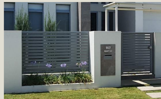
3.4.1 Spacing width between palings less than 50% of the paling width
